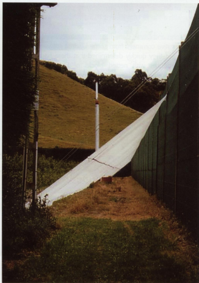
Barnes Deflection Shelter
