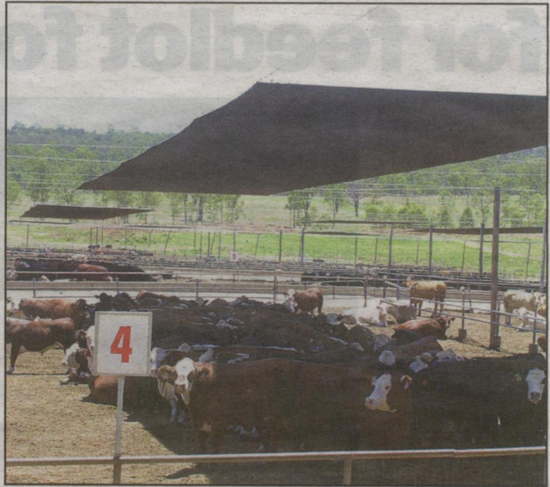
The high tension cabling systems used to support shade cloth at Maydan largely do away with the need for internal posts.
