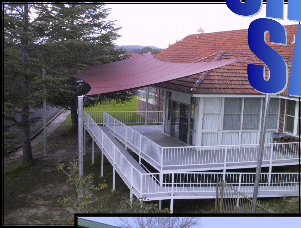
Local Hospital - Recreation/entrance Area
