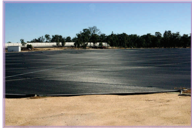
Below: Dam Cover constructed at wall height reduces wind loads.
